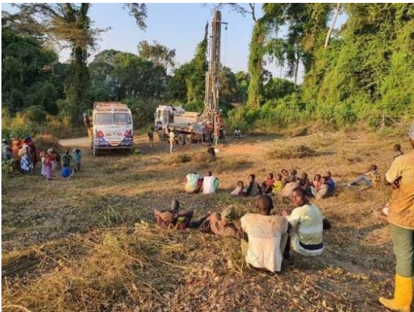
Initiation of borehole construction
